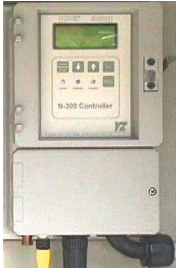
↑ I.S. Power Supply Connection
